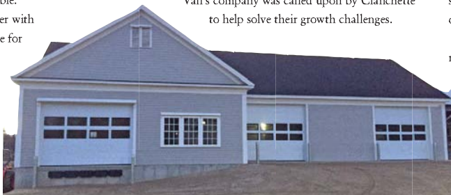
The new Main Line Fence workshop features interior and exterior eastern white pine sheathing, which contributes significantly to the energy efficiency of the structure.
